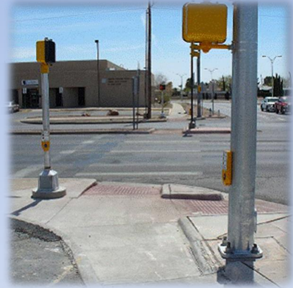
Example of ADA compliant pedestrian accommodations
