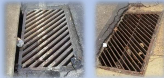
Existing Drainage Grates
