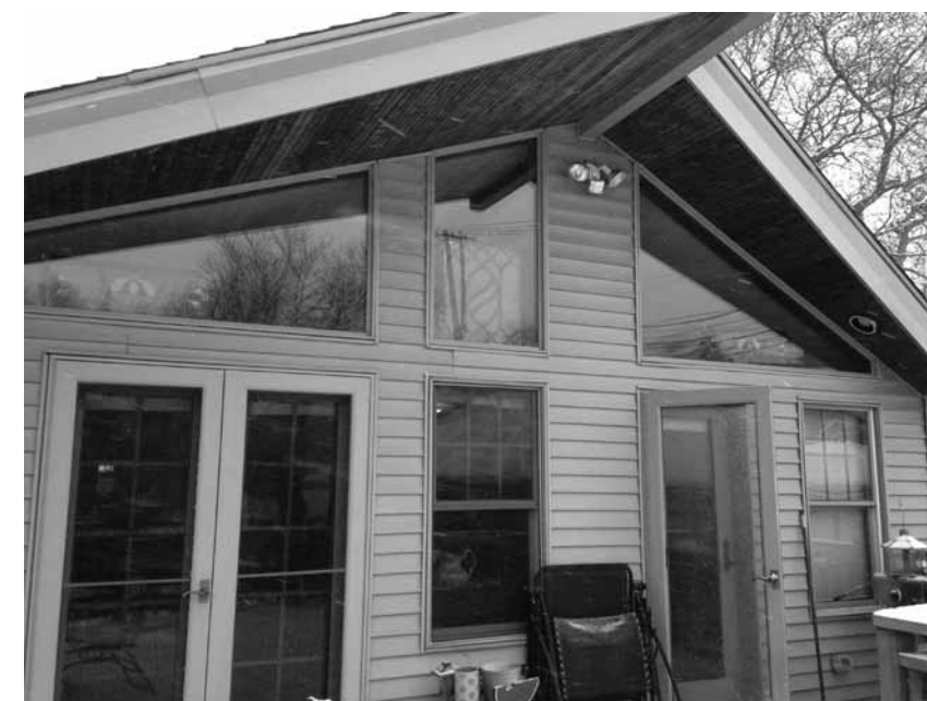
Work completed by Kramer Construction
